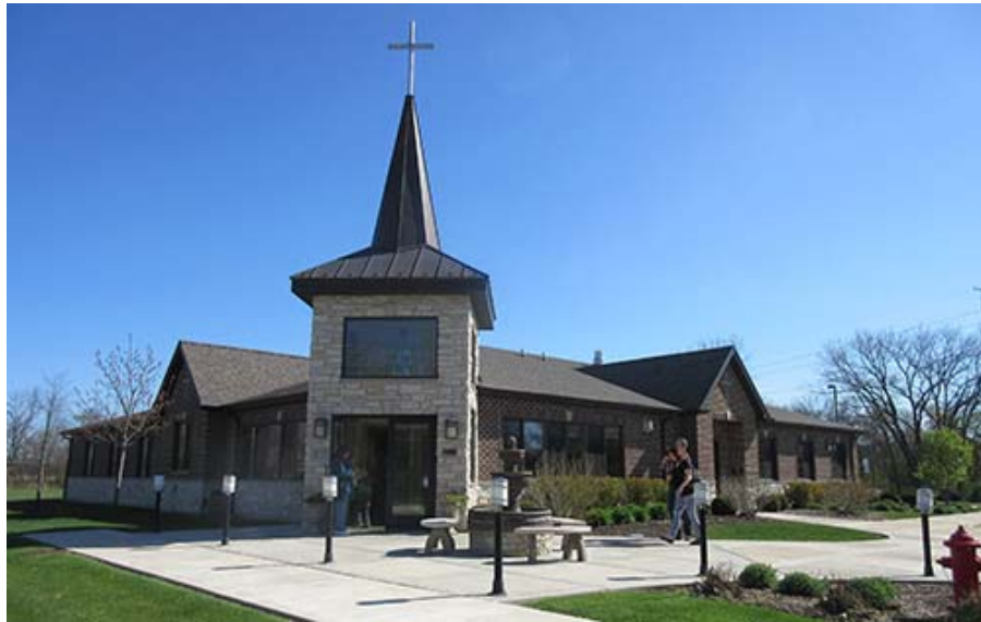
The LifeSpring facility
