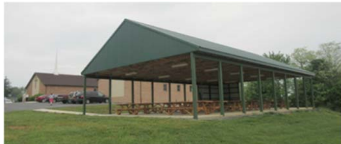
New pavilion at the Mt Holly Springs church
